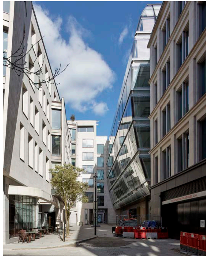
Transformation of New Burlington Place view looking east
