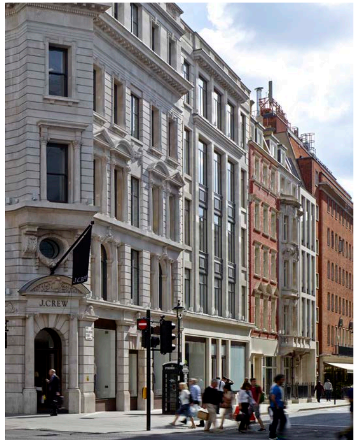
Transformation of New Burlington Street, May 2014
