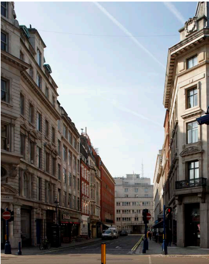
Existing view of New Burlington Street, May 2009
